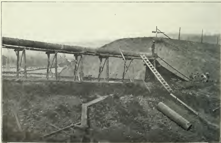
FIG. 2.—LAKE FRANCES DAM. SLICING ON THE BREAK APPROACHING THE TOP.
