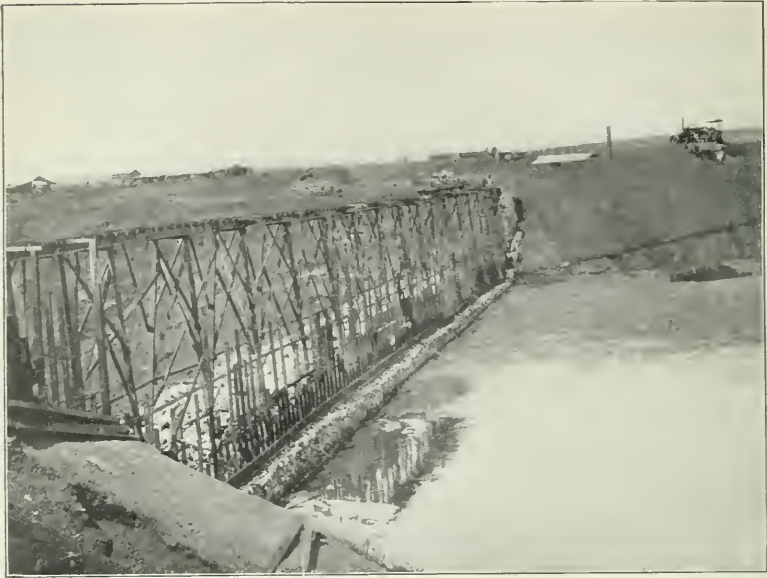
FIG. 1.—WAIALUA DAM. SHOWING HYDRAULIC FILL BEING SLICED IN AGAINST THE ROCK-FILL.
