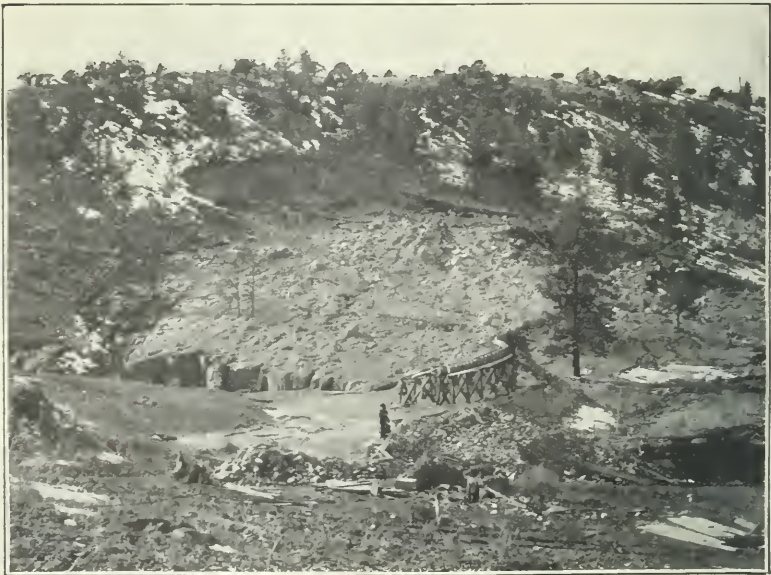
FIG. 2.—TERRACE DAM. DEPOSIT OF HYDRAULIC FILLING ON THE UPPER TOE SLOPE.
