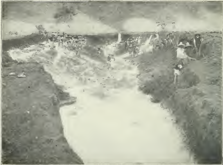
FIG. 1.—GROUND-SLICING ON DAM NO. 1. TENANGO RIVER.
