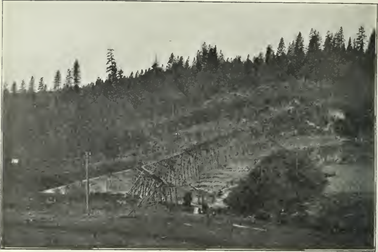
FIG. 1.—LAKE FRANCES DAM. JANUARY 29TH, 1902. TRESTLE NO. 5. 1 150 FT. LONG; DISCHARGE END AT ELEVATION 59 FT. ABOVE DATUM.
