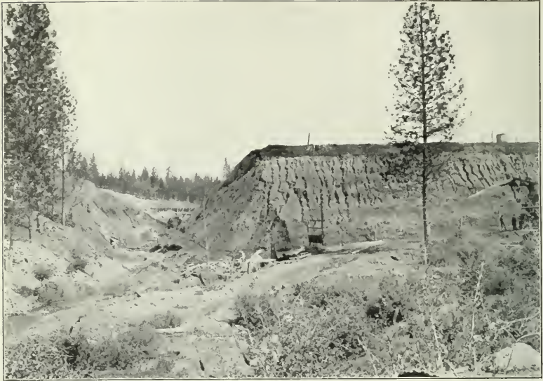
FIG. 1.—BREAK IN ORIGINAL LAKE FRANCES DAM. LOOKING UP STREAM.
