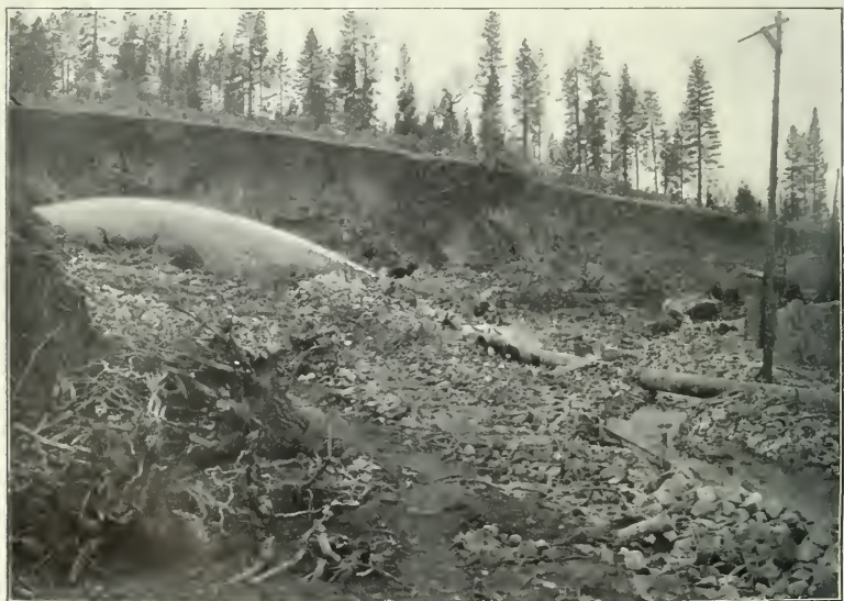
FIG. 2.—HYDRAULIC GIANT IN ACTION UNDERCUTTING THE BANK.
