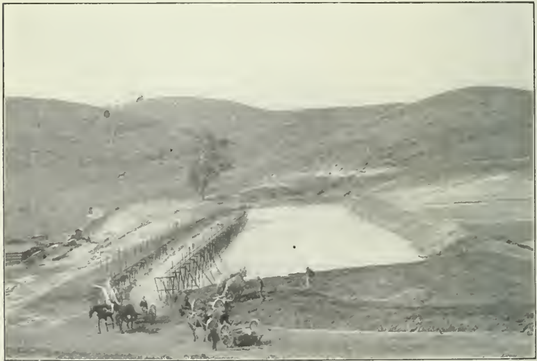
FIG. 2.—SILVER LAKE DAM, WITH LEVEES BUILT UP DRY WITH SCRAPER TEAMS.
