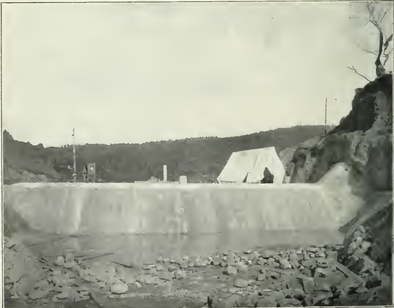
FIG. 2.—SPILLWAY OF LAKE FRANCES DAM, 80 FT. LONG. THE WATER-CUSHION IS 5 FT. DEEP.
