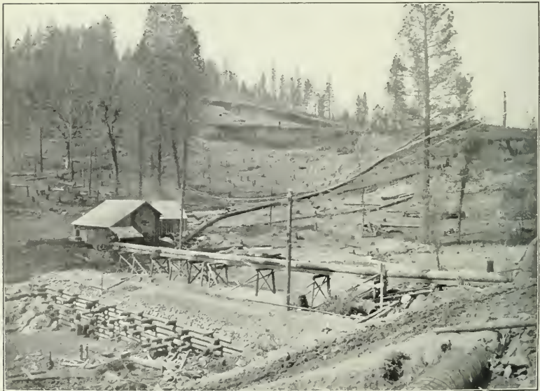
FIG. 2.—LAKE FRANCES DAM CONSTRUCTION. PUMPING STATION. SHOWING SUCTION PIPE CONNECTED TO TANDEM CENTRIFUGAL PUMP. CRIB DAM IN FOREGROUND BUILT TO STORE WATER FOR EARLIER OPERATIONS.
