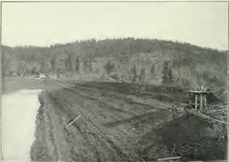
FIG. 2.—LAKE FRANCES DAM COMPLETED. SHOWING THE TOP OF THE BURIED GATE TOWER ON THE SIXTEEN-INCH OUTLET.
