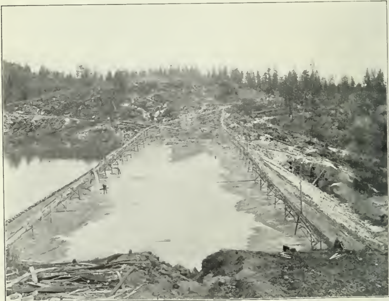
FIG. 2.—CRANE VALLEY DAM, NEARING THE 70-FT. LEVEL, WHERE SLICING OPERATIONS CEASED.
