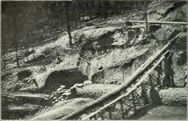
FIG. 1.—LAKE FRANCES DAM. SLUICING PLANT USED WITH SIX-INCH CENTRIFUGAL PUMP FOR FILLING THE BREAK.
