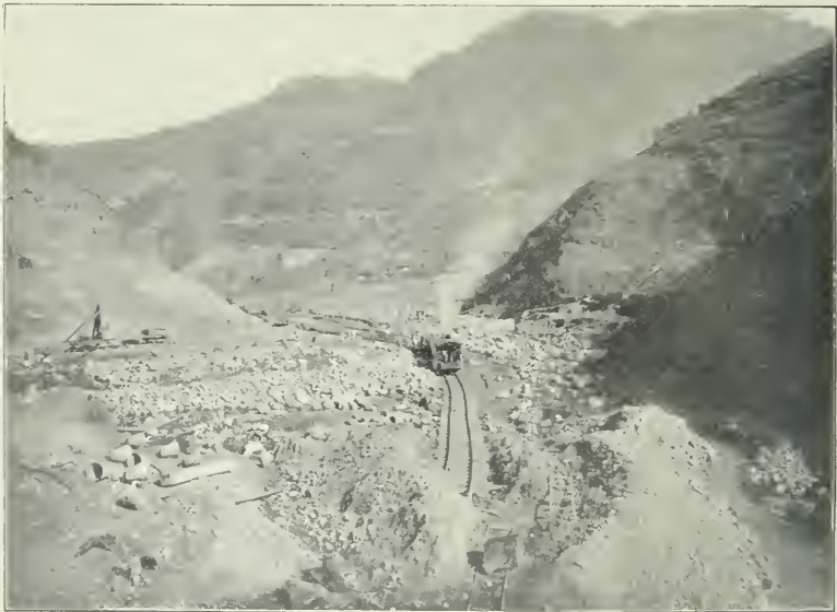
FIG. 2.—LOOKING UP STREAM AT SITE OF DAM No. 2, AT NECAXA. SHOWING STRIPPED ABUTMENTS FOR THE DAM ON EACH SIDE.
