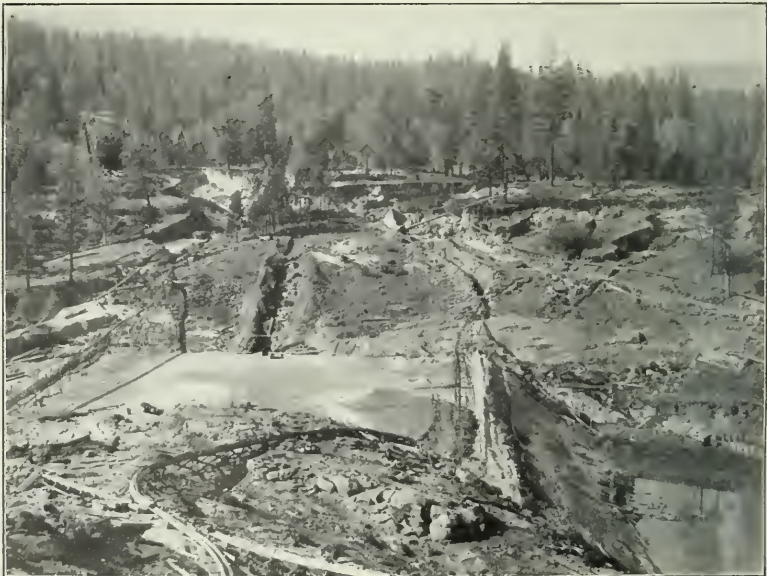
FIG. 2.—BORROW-PITS FROM WHICH MATERIAL WAS SLICED TO THE CRANE VALLEY DAM.
