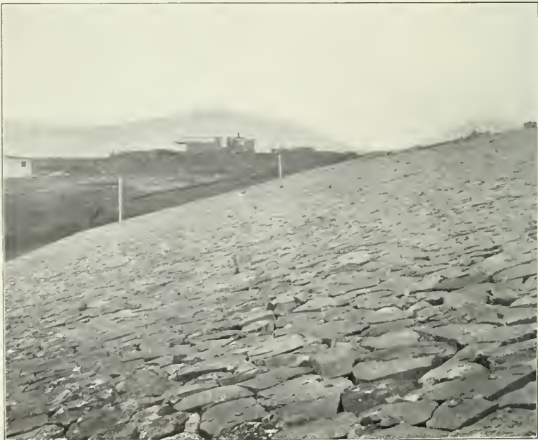
FIG. 2.—RIP-RAP ON FACE OF HYDRAULIC-FILL, WAIALUA DAM.
