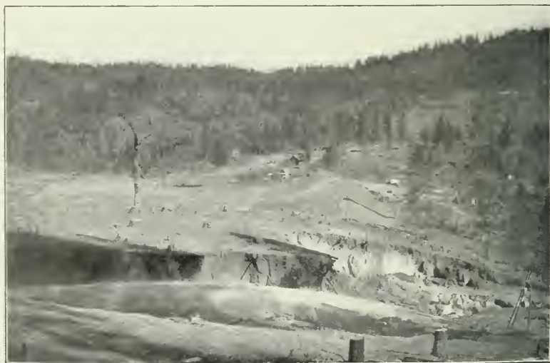
FIG. 2.—LAKE FRANCES DAM, NOVEMBER 6TH, 1901. FROM SOUTH BORROW-PIT, LOOKING ALONG AXIS OF ORIGINAL DAM.
