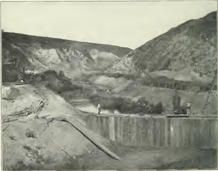
FIG. 2.—WAIALUA DAM SITE. LOOKING DOWN STREAM. SHOWING THE GORGE FILLED BY THE DAM.
