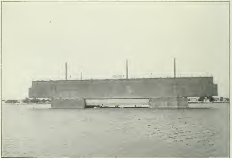
FIG. 2.—SELF-DOCKING: SIDE VIEW, SHOWING CENTER PONTOON DOCKED.
