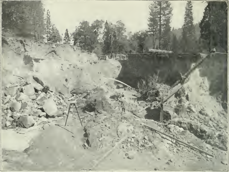
FIG. 1.—CRANE VALLEY HYDRAULIC-FILL DAM. SHOWING METHOD OF LOOSENING THE MATERIALS SLICED INTO THE DAM.
