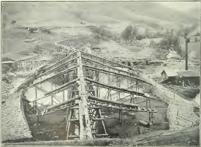
FIG. 2.—DAM NO. 1 ON THE TENANGO RIVER. LOOKING NORTH.
