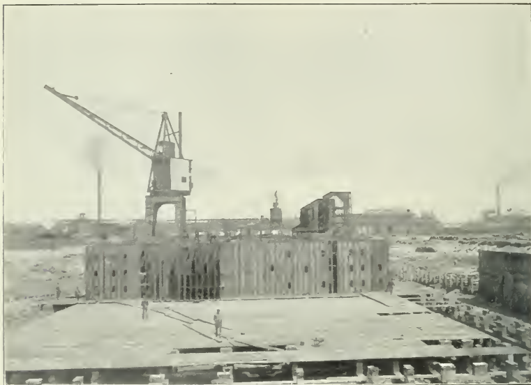
FIG. 1.—VIEW OF DOCK, MAY 1ST, 1904; BOTTOM PLATING AND BOW PONTOON IN POSITION.
