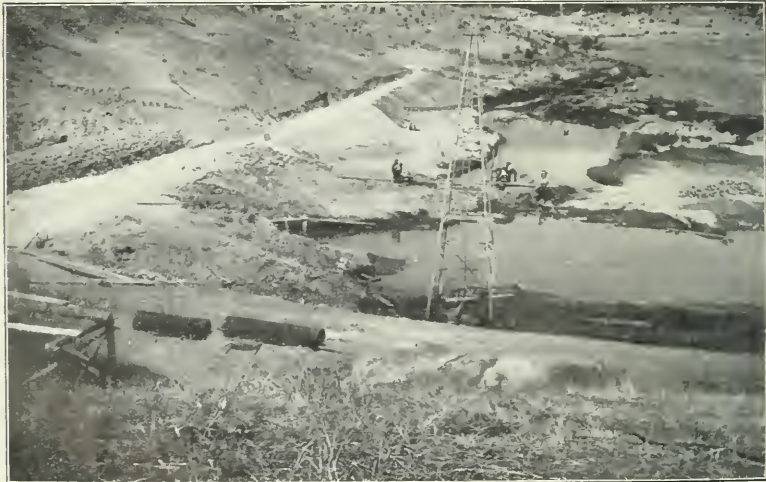
FIG. 2.—LAKE FRANCES DAM. LOOKING UP INTO THE RESERVOIR FROM THE TOP OF THE ORIGINAL DAM. AUGUST 31ST, 1901.
