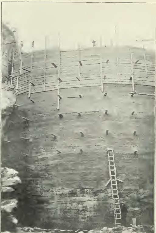
FIG. 1.—UP-STREAM SIDE, CONCRETE CORE-WALL TERRACE DAM.
