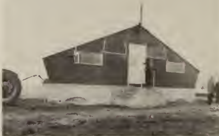
The new feeder hog building.
